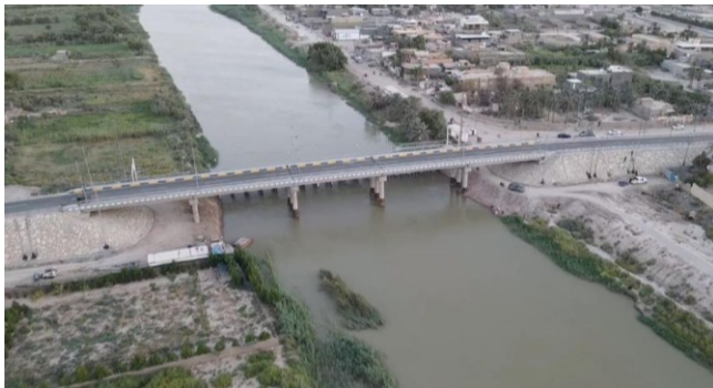
Fig 4. A picture of the bridge structure showing the abutments and embankments.
